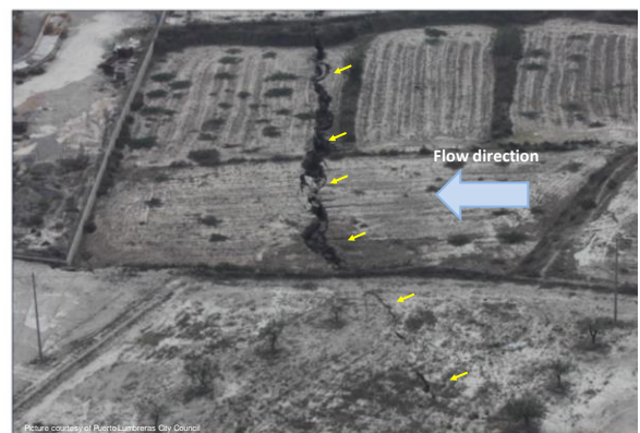
Figure 5: Aerial view of the 3 rd and 2 nd northern section of the crack (courtesy of Puerto Lumbreras City Council). The yellow arrows indicate the location of the earth fissure. Modified from Mulas (2013).
