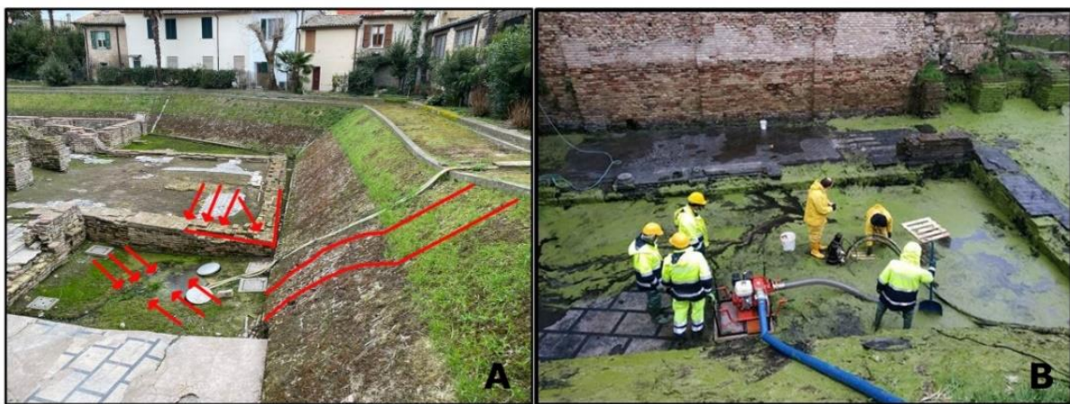
Figure 2A Land settlements and instability of the soil slope and of the old brick masonry walls, concentrated around the tank area. B) Drainage operations by Civil Protection of the flooded Archaeological Area of Santa Croce as a consequence of the temporary break down of the pumps (August 2021).
