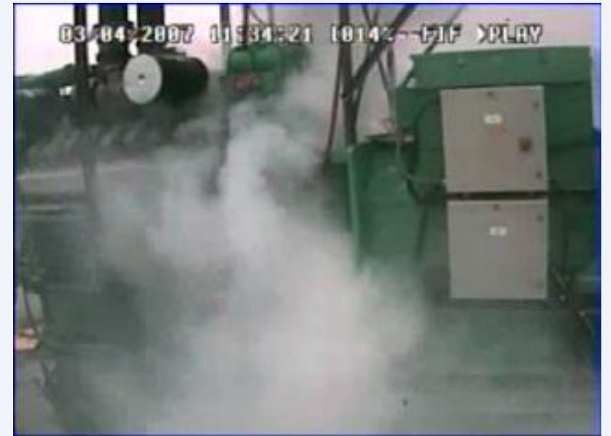
Idaho Labs, 2007: disable power plant through cyberattack
