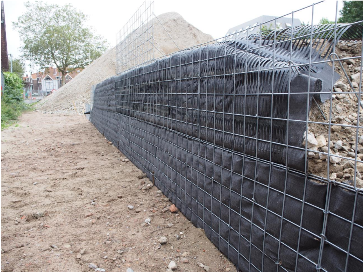
Fig. 6. Temporary support of the vertical slope
