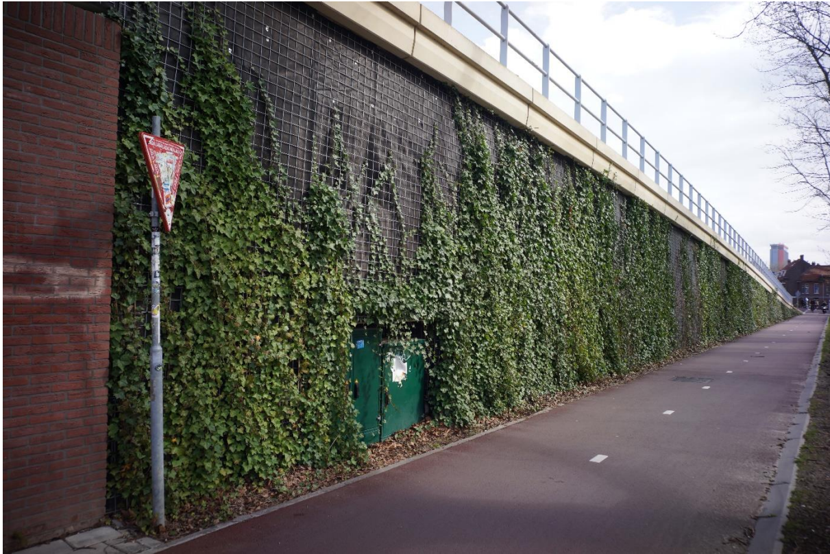
Fig. 9. Access ramp south bank (west side) final result
