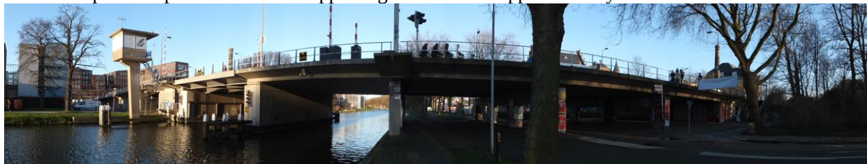
Fig. 1. Panoramic overview of the old bridge
